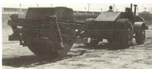
Figure 1. The impact roller about to deliver a blow.
