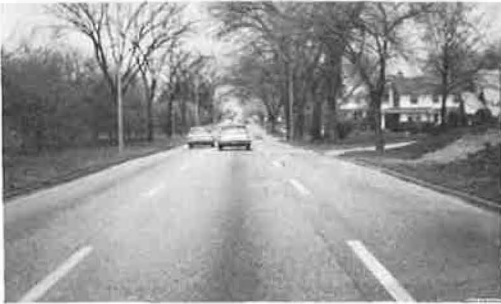
Figure 9. Typical view on Ward Parkway.
