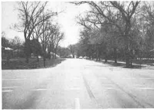
Figure 7. Southward view on Ward Parkway at Meyer Boulevard.
