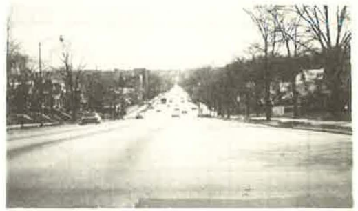
Figure 12. Typical view on The Paseo.
