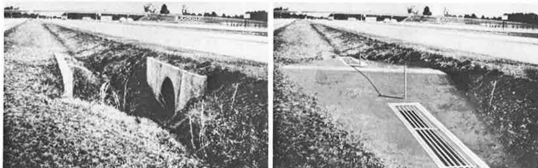
Figure 4. Modification of existing culvert crossover with headwalls (1).
