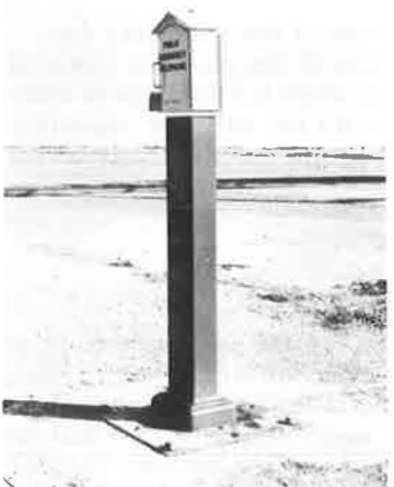
Figure 3. Ohio call-box assembly.
