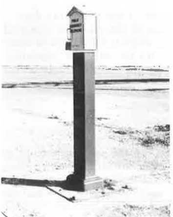
Figure 3. Ohio call-box assembly.
