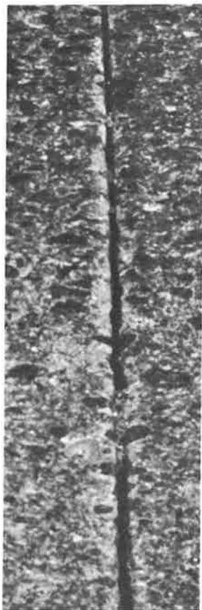
Figure 25. Polysulfide-sealed joint (truck lane).
