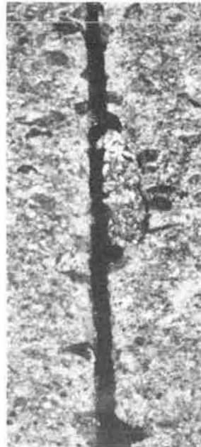
Figure 31. Close-up of polysulfide-sealed joint (truck lane).
