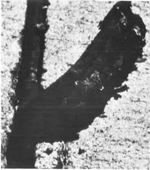
Figure 5. Polysulfide seal with embedded debris.
