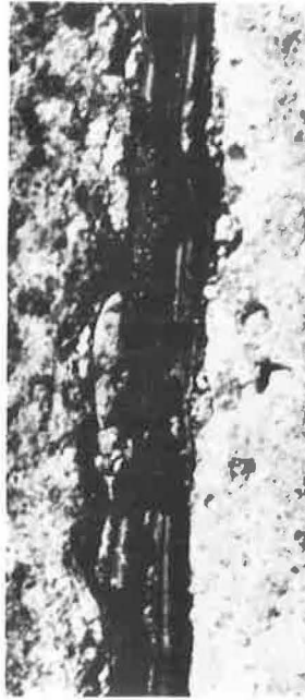
Figure 40. Close-up of core area (neoprene-sealed joint).
