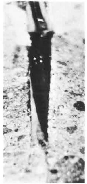
Figure 41. Undamaged core area (neoprene-sealed joint).
