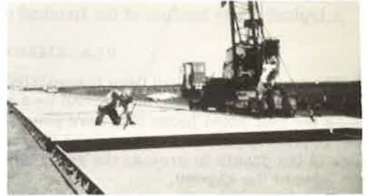
Figure 6. Placing panels in the west section.
