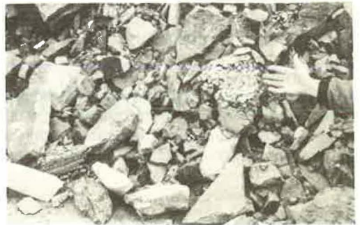
Figure 9. Typical massive deterioration of argillaceous dolomite with rejection texture.
