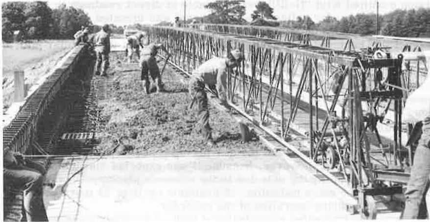
Figure 1. Longitudinal bridge deck screeding machine.
