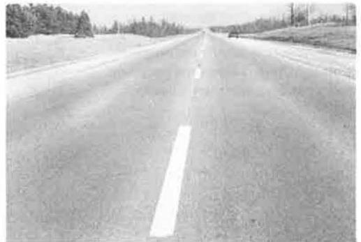
Figure 8. Four-year old pavement made with 150- to 200-penetration asphalt.
