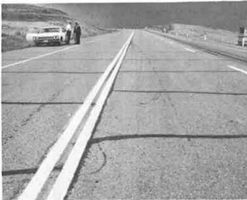
Figure 5. Typical low-temperature transverse pavement cracking (4-year old pavement made with 150- to 200-penetration asphalt).
