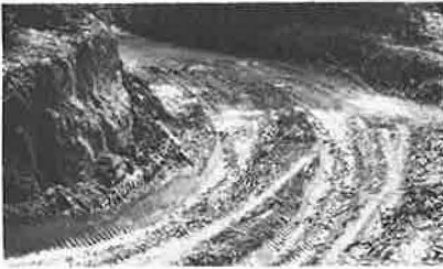
Figure 6. Deep rutting in Virginia road.
