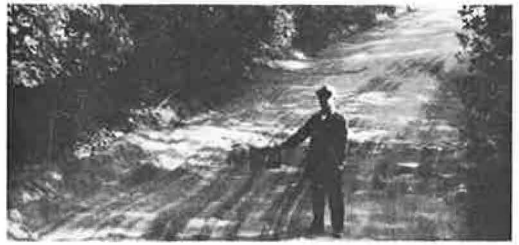
Figure 5. Deep depressions in Virginia road.
