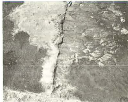
Figure 6. Channels indicating water movement on CTB surface.
