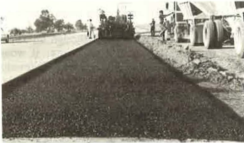
Figure 3. Rolling of permeable AC, US-99.
