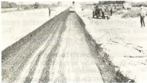
Figure 3. Rolling of permeable AC, US-99.
