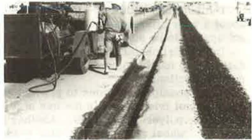
Figure 4. Partial shoulder replacement, I-80.
