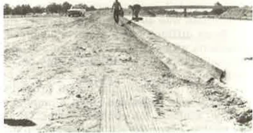
Figure 2. Fiberglass-reinforced plastic placement, US-99.
