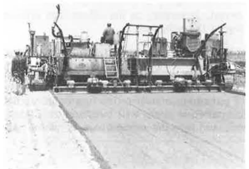
Figure 7. Placing CTB with slip-form paver.
