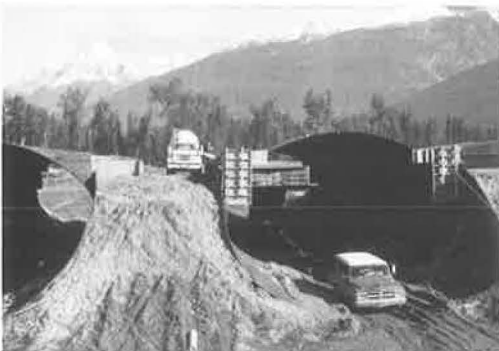
Figure 23. Large culverts in British Columbia (furnished by Chriss Fisher, Armco Corporation).
