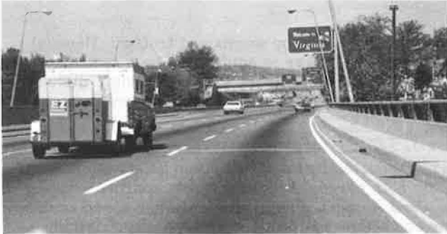
Figure 2. Limited sight distance on the approach to exit 1.
