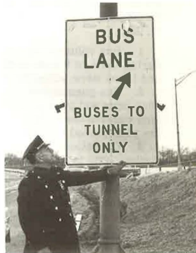
Figure 5. Police officer activating hinged, changeable bus lane guide sign.
