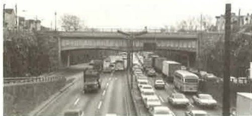
Figure 3. Overhead lane directional signals and plastic traffic posts to separate exclusive bus lane from westbound flow.
