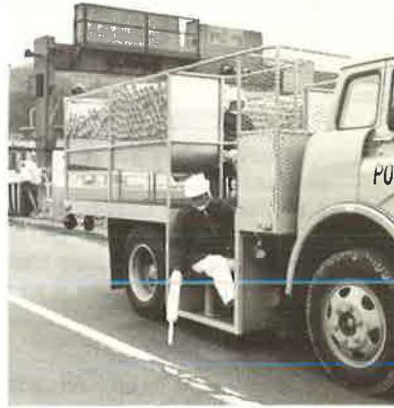
Figure 4. Port Authority personnel in specially equipped vehicle inserting plastic traffic posts into pavement holes.
