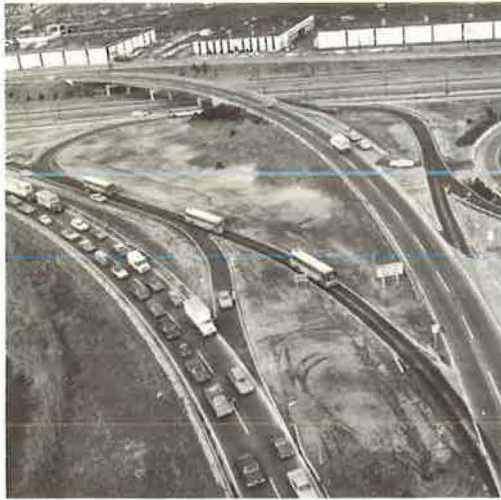
Figure 2. Bus access roadway at New Jersey Turnpike interchange; exclusive bus lane entrance at lower right. "Escape hatch" roadway at center allows off-route vehicles to enter regular eastbound flow.
