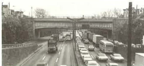
Figure 3. Overhead lane directional signals and plastic traffic posts to separate exclusive bus lane from westbound flow.
