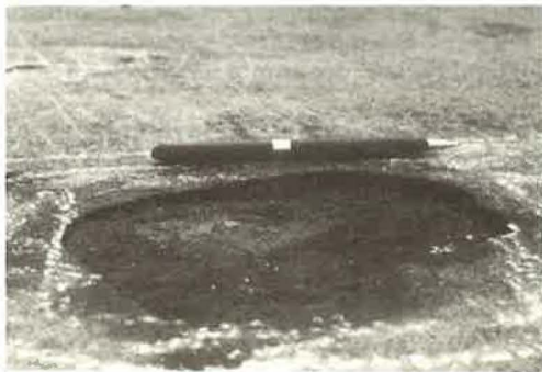
Figure 6. Example of 1/4- to 1/2-in. deep spall.
