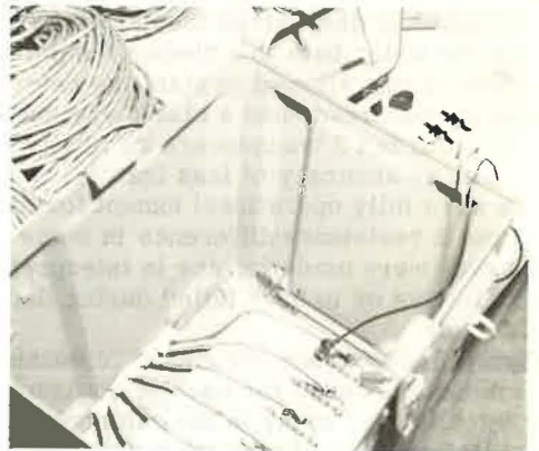
Figure 4. Terminals in junction box.
