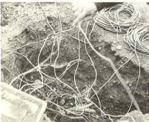
Figure 7. Wired system during placing in shoulder area.
