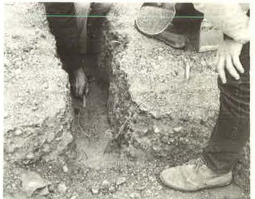
Figure 6. Transducers being buried in shoulder area beneath subbase.
