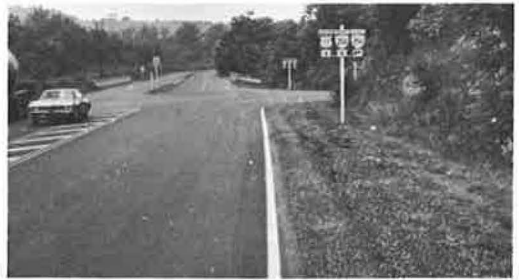
Figure 10. Bridge located at end of pavement transition from two to four lanes.
