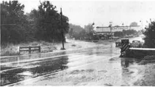
Figure 9. Bridge with narrow roadway located adjacent to intersection (center) and business entrance (right foreground).
