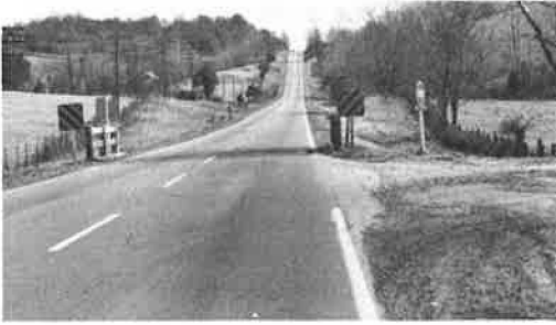
Figure 2. A narrow bridge located within a passing opportunity section of two-lane highway with intersection to the right adjacent to the structure.
