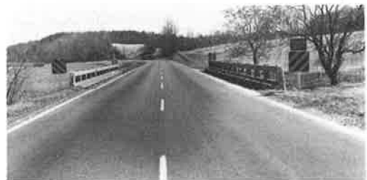
Figure 6. Restricted roadway width and exposed ends of rigid concrete railing.
