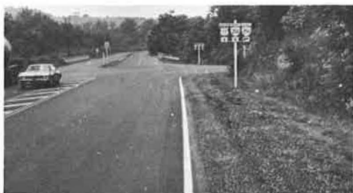
Figure 10. Bridge located at end of pavement transition from two to four lanes.
