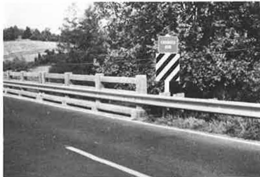
Figure 8. Approach guardrail continued across a bridge.
