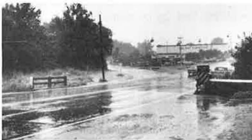
Figure 9. Bridge with narrow roadway located adjacent to intersection (center) and business entrance (right foreground).
