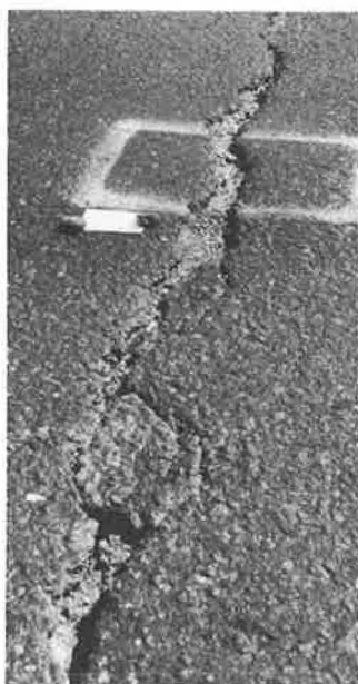
Figure 5. Wide transverse crack in asphalt pavement over contraction joint in reinforced concrete base (section G).
