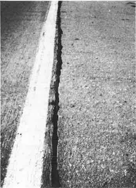
Figure 1. Sealed joint on I-80 in Illinois after 5 years of service.
