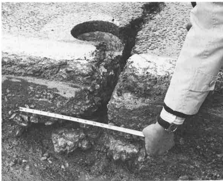
Figure 7. Severe spalling in bottom half of concrete base slab at wide crack (section D).
