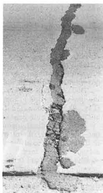
Figure 6. Wide stepped transverse crack, about 3½ in. wide, in continuously reinforced concrete pavement (section H).
