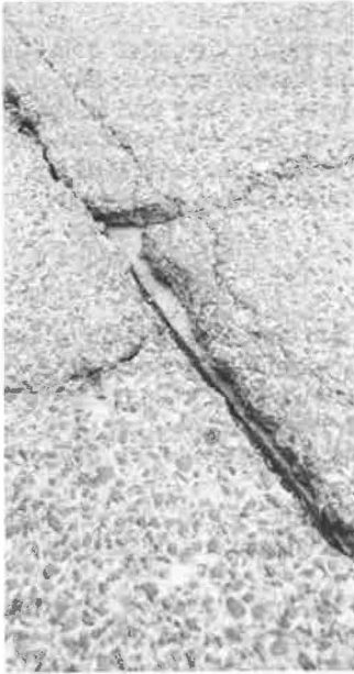
Figure 9. Loss of asphalt pavement due to cracking at centerline joint (section D).
