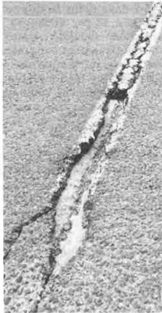
Figure 10. Loss of asphalt pavement due to cracking at centerline joint (section F).
