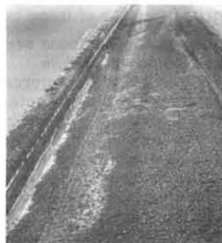
Figure 13. Surface water in granular shoulder at edge of pavement.
