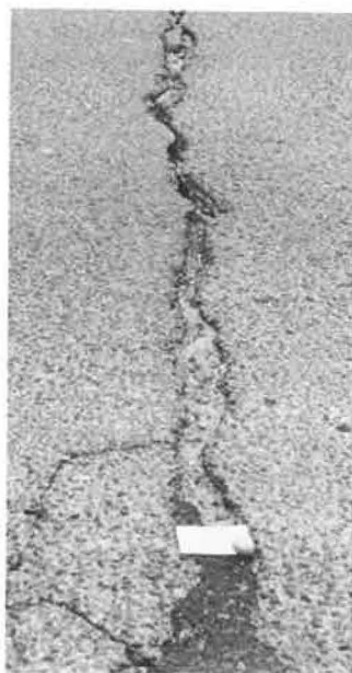
Figure 4. Wide transverse crack in asphalt pavement on unreinforced concrete base (section A).
