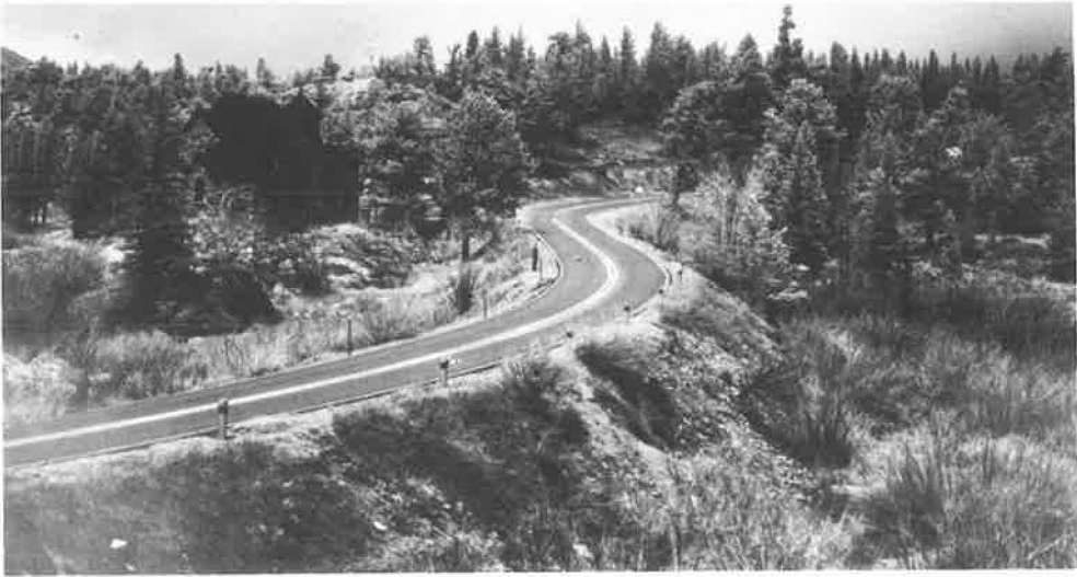
Figure 1. Photograph of existing terrain and old highway, Colo-7.
