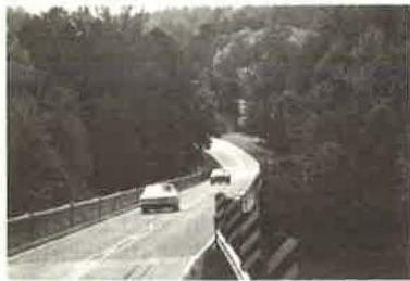
view looking west—Haw River Bridge
