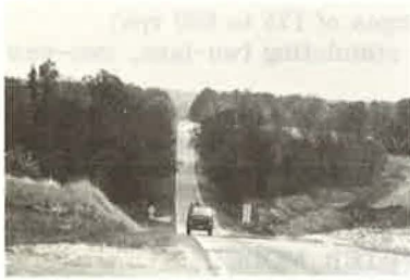
view looking east—restriction 1(V)
