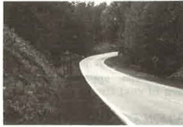
view looking west—restriction 3(H)
