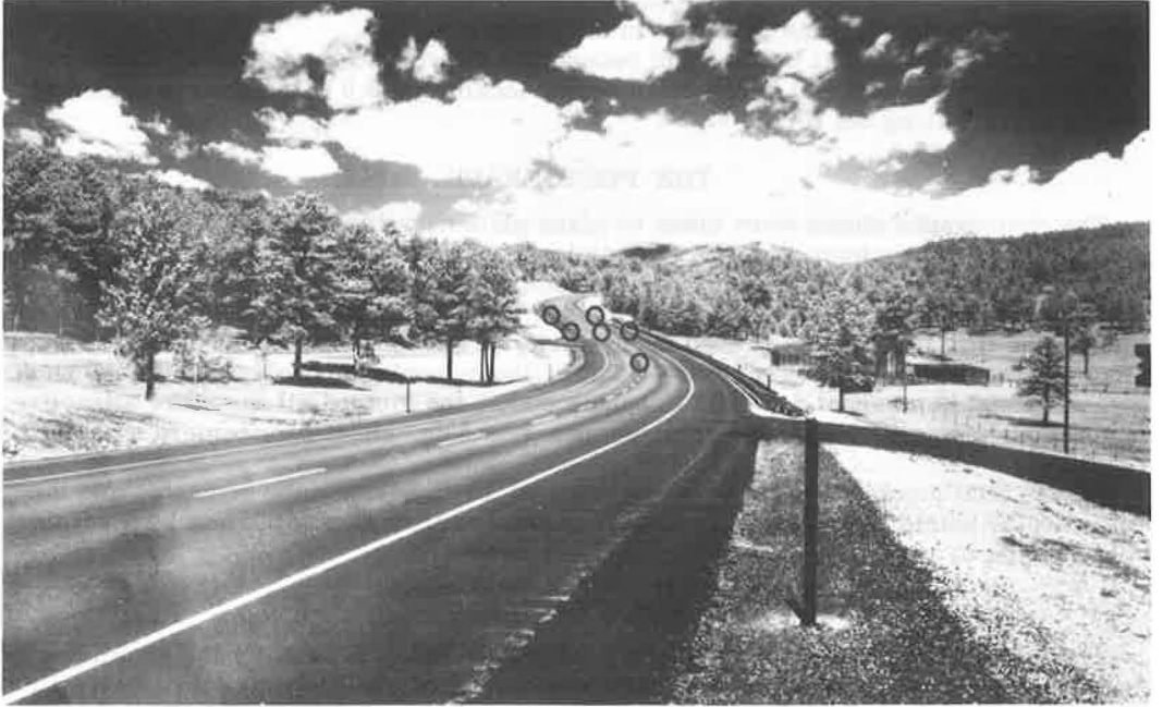
Figure 6. Photograph of existing highway with resectioning points.
