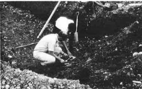
Figure 11. Sensor installation in trench.
