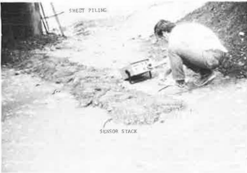
Figure 6. Covered sensors and cables before deposit of loose lift.
