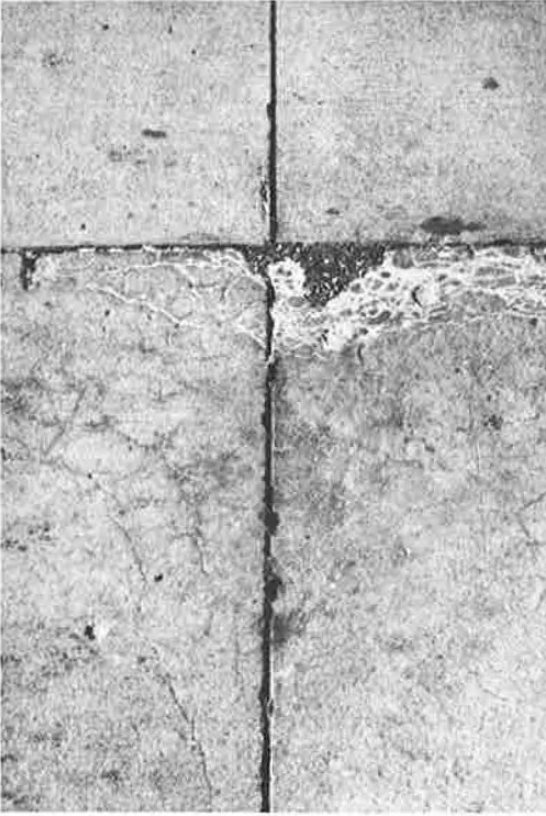
Figure 6. Typical D-cracking along a transverse joint in the Topeka test road, where 1½-in. maximum-sized aggregate particles were used.
