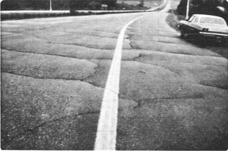
Figure 10. Polygonal cracking.
