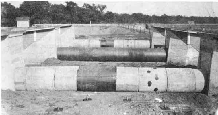
Figure 6. Experimental culverts before fill construction.
