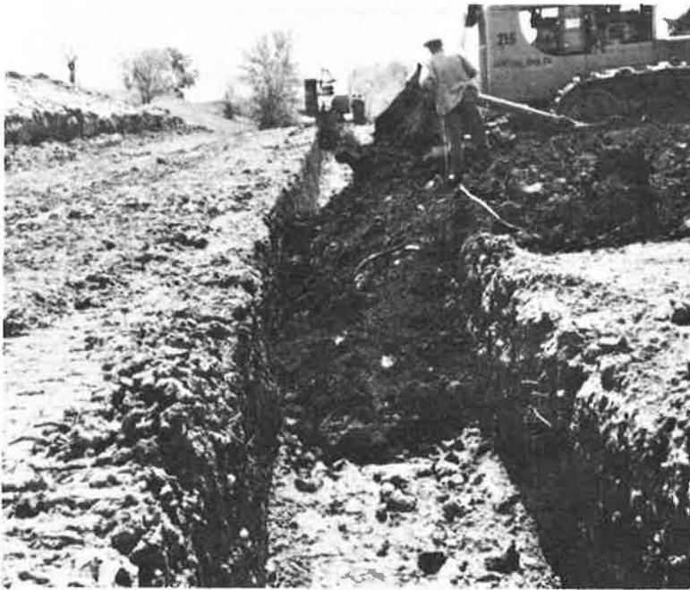
Figure 7. Refilling trench with compressible material.
