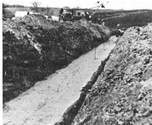
Figure 6. Six-inch compacted sand bed.
