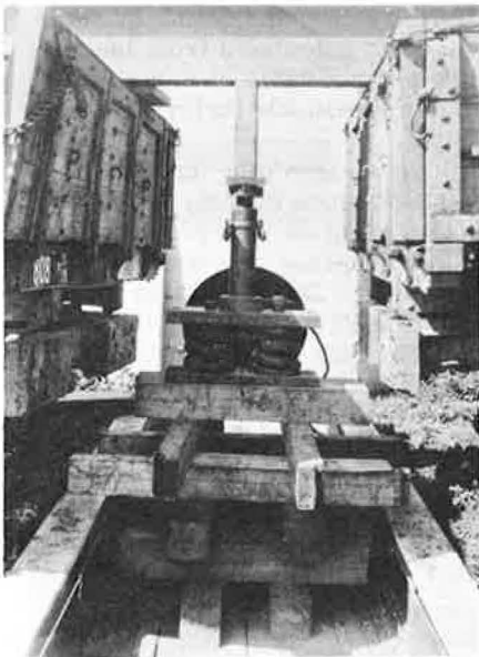
Figure 9. Weighing platforms calibrated by hydraulic jack and spring-bearing arrangement.
