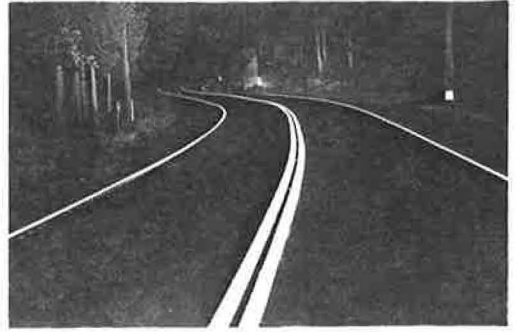
Figure 2. Same road as shown in Figure 1 after being striped with yellow lines at center and white lines at edge.
