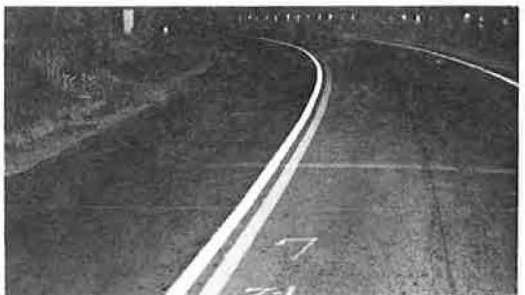
Figure 5. Standard reflectorized line (left) and nonreflectorized line (right).
