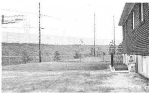
Figure 8. Highway 401 noise barrier.
