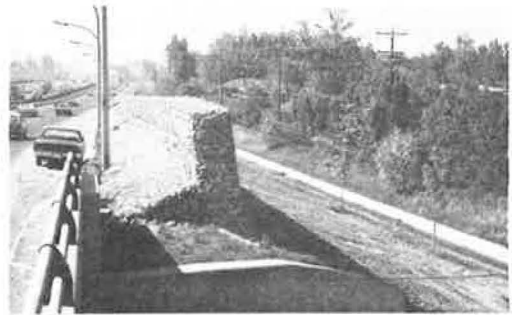
Figure 9. Gabion wall, Don Valley Parkway.
