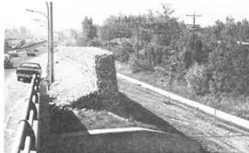
Figure 9. Gabion wall, Don Valley Parkway.
