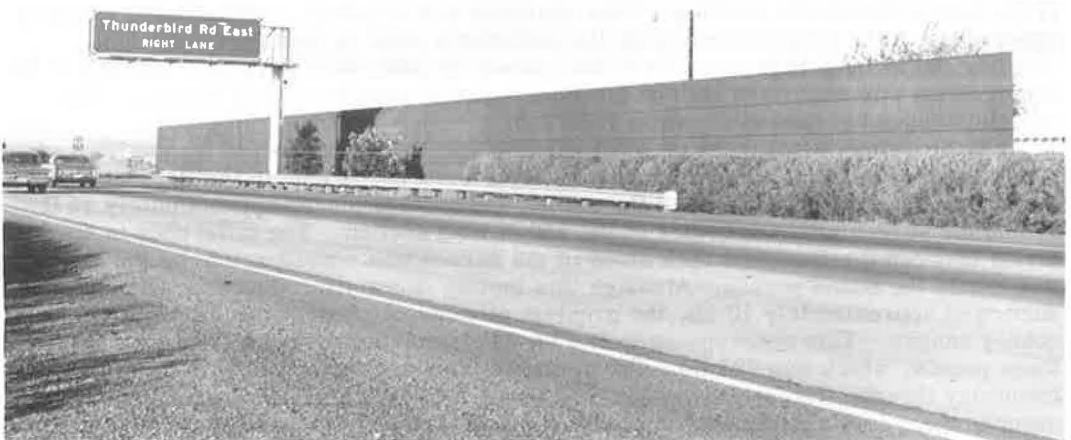
Figure 9. Full-scale Kinematic Sound Screen (aluminum construction).
