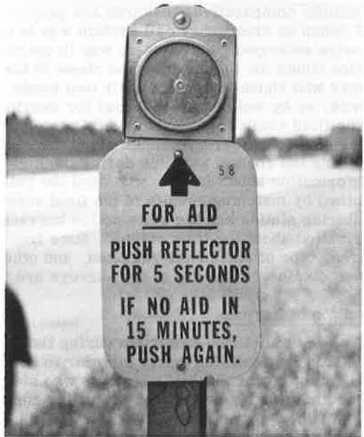
Figure 1. Reflective push-button switch: call station.
