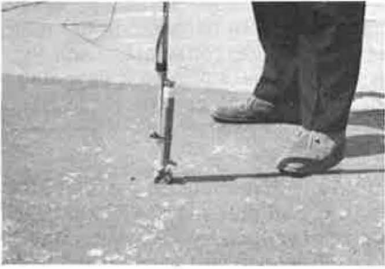
Figure 6. Measuring electrical potentials between a copper-copper-sulfate half-cell and the steel reinforcement.
