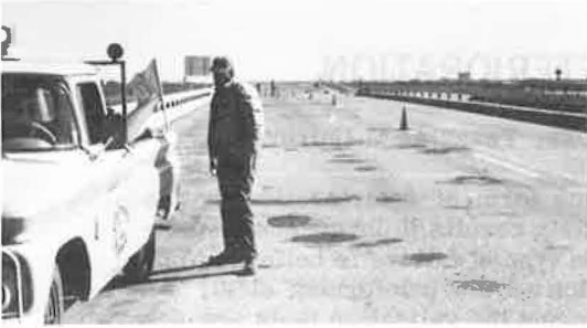
Figure 1. Delamination repair.
