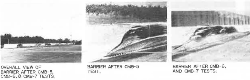
Figure 12. CMB barrier damage.
