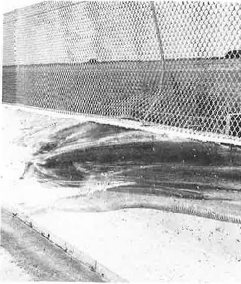
Figure 15. Damage to CMB-2.
