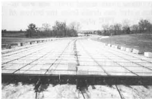
Figure 1. Plastic-coated tendons and bulkhead beam with dowels in place.
