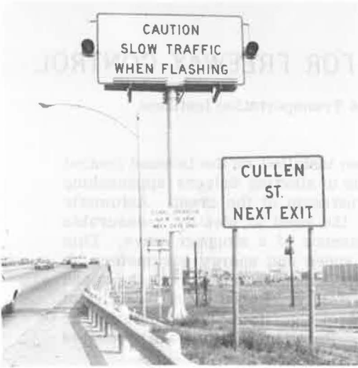
Figure 1. Warning sign with flashers.
