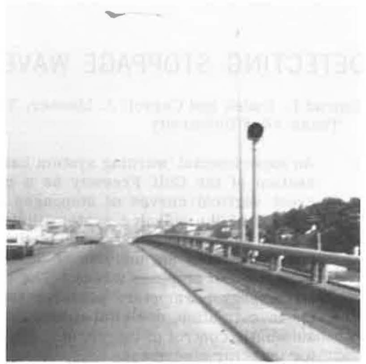
Figure 2. Flasher unit at crest of overpass.
