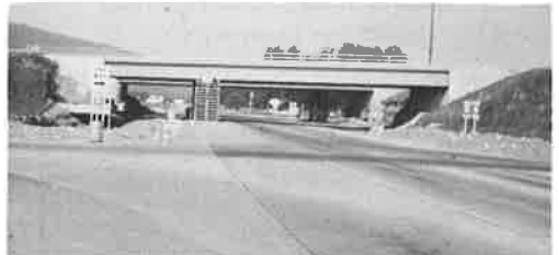
Figure 11. Timber cribbing supporting US-17 interchange bridge until abutments could be underpinned.
