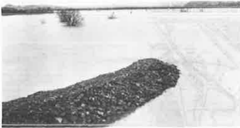
Figure 14. Rockfill spur dike near Susquehanna River bridge in Nanticoke, Penn., during 1964 flood.
