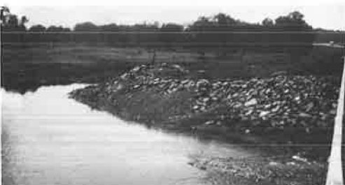
Figure 16. Remnants of earthfill spur dike near Chemung River bridge near Lowman, N.Y.
