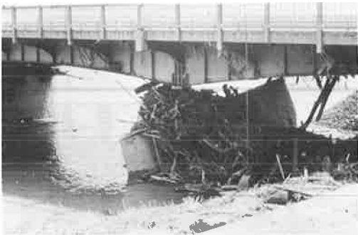
Figure 13. Settlement due to scour on Chemung River bridge in Elmira, N.Y.
