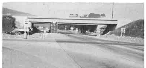
Figure 11. Timber cribbing supporting US-17 interchange bridge until abutments could be underpinned.
