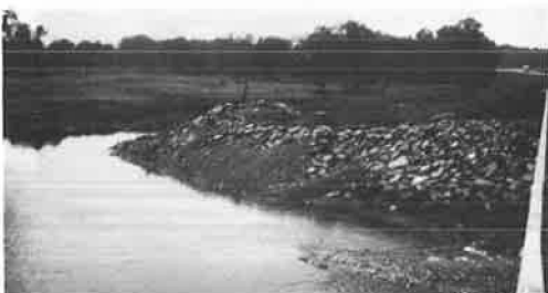
Figure 16. Remnants of earthfill spur dike near Chemung River bridge near Lowman, N.Y.
