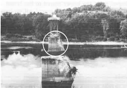
Figure 5. Post-flood remnants of the James Street bridge.
