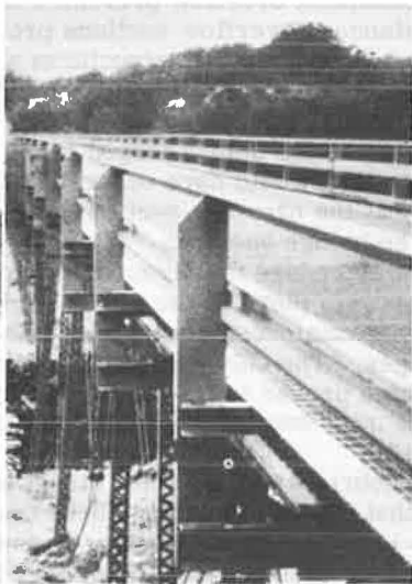
Figure 6. Exposed piling and undermined abutment of Chemung River bridge.
