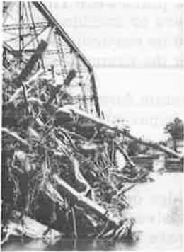
Figure 1. Debris deposited on bridge by floodwaters.
