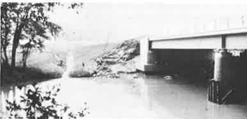
Figure 10. Upstream view of scoured bridge abutment and approximately 2 ft of exposed piling on Canisteo River bridge.
