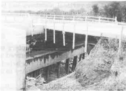
Figure 6. Exposed piling and undermined abutment of Chemung River bridge.
