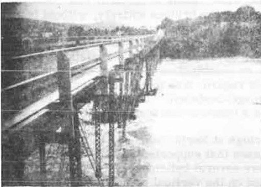
Figure 5. Post-flood remnants of the James Street bridge.
