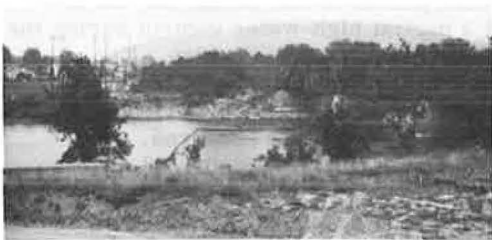
Figure 19. Upstream scour hole, eroded approach embankment, and damaged abutment of Lehigh Valley Railroad bridge.
