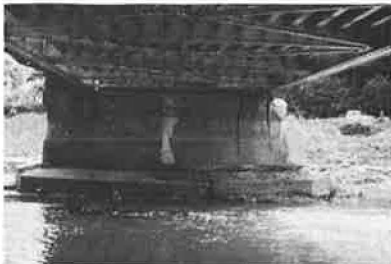
Figure 23. Cracked pier shaft supporting a county bridge on Schrader Branch of Towanda Creek.
