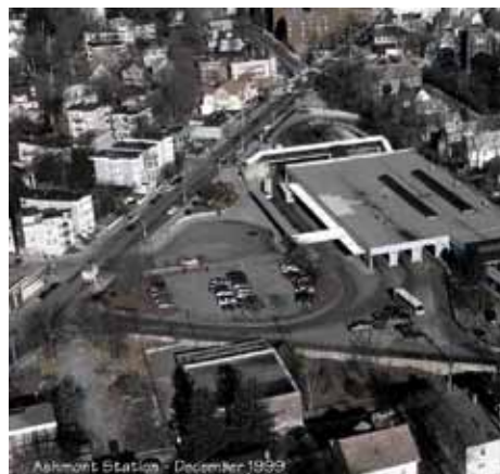
Ashmont Station before improvements. A PCC is visible on the viaduct (lower right). This viaduct, which crosses the "heavy rail" Red Line tracks, was removed and reconstructed, necessitating a service shutdown. (Photo: MBTA)
