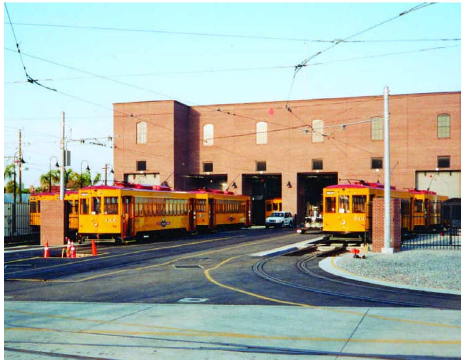
The full carbarn, located on Nuccio Parkway between Sixth and Seventh Avenues, before the fleet of “new” cars start morning service.
