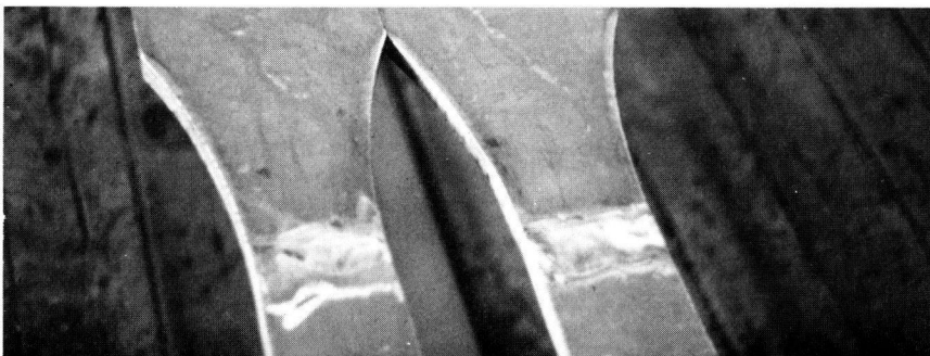
Figure C-8. Weld reinforcement removed by grinding and transition given final shaping.
