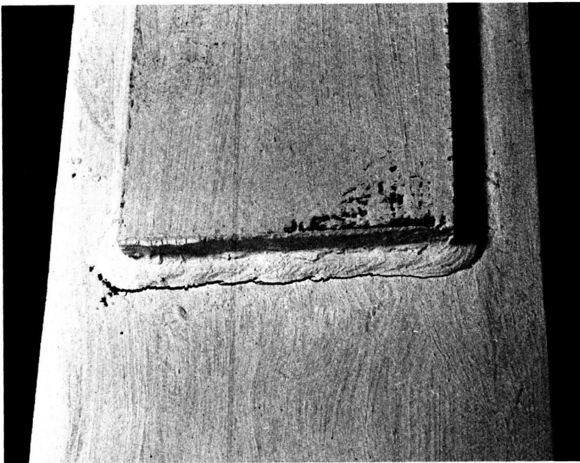
Figure 12. Crack formation at toe of transverse fillet weld.
