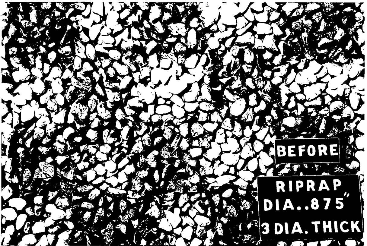
Figure 59. The layer of riprap on the 4:1 side slope is the equivalent of three grain diameters thick. With such placement the base material is apparently well protected and safe from turbulent eddies that seek to penetrate the riprap. The surface was sprayed with paint in the form of a grid to assist in locating the same point after the experiment
