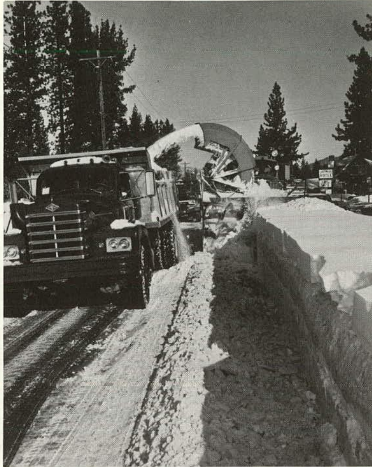
BLOWER LOADING SNOW FOR REMOVAL FROM TEMPORARY STORAGE
