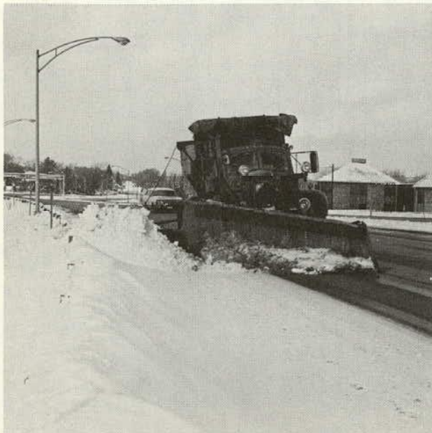
Figure 19. Wing plow clearing snowdrifts from shoulder.
