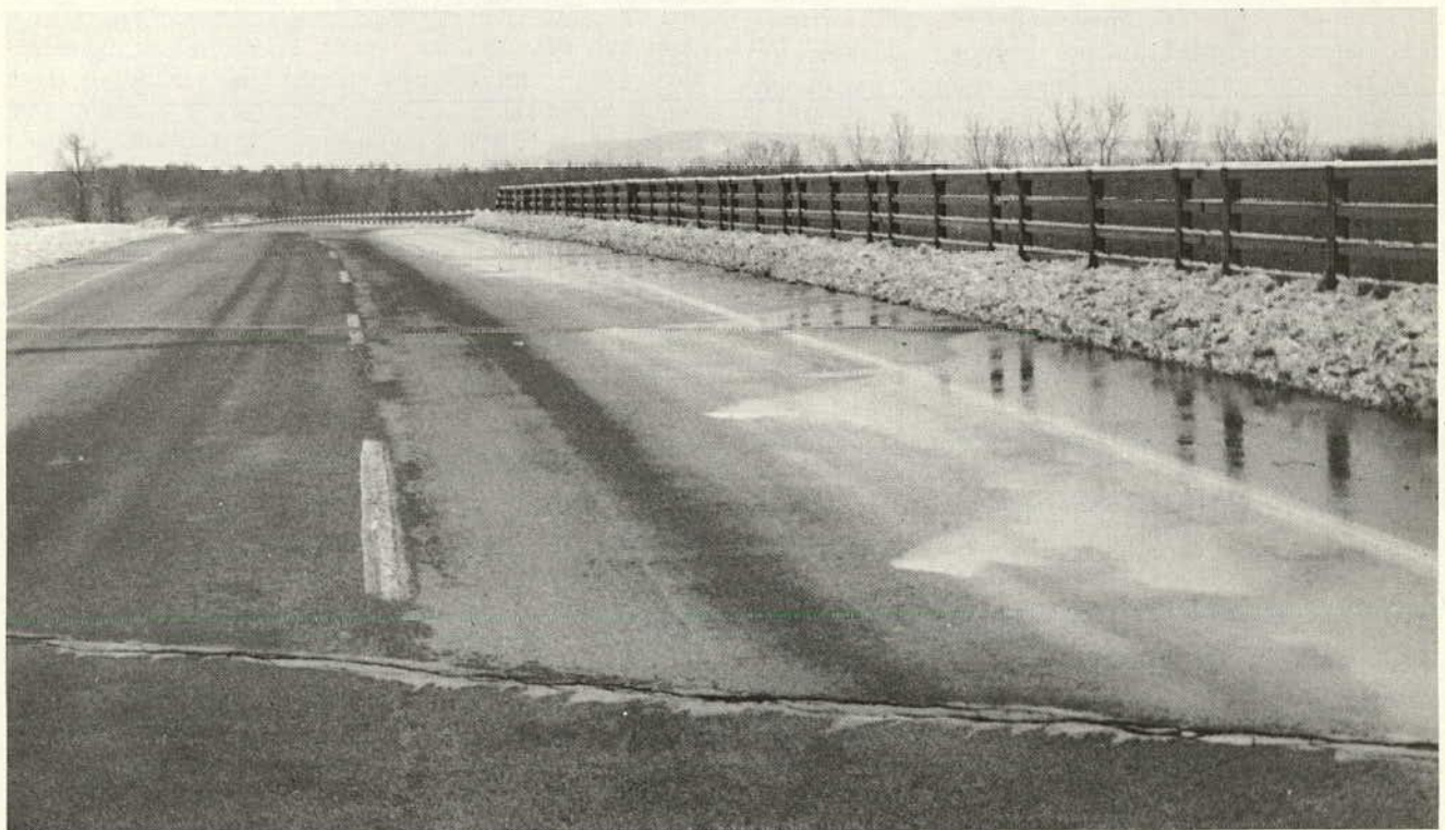
Figure 6. Melt water on bridge deck subject to refreezing.
