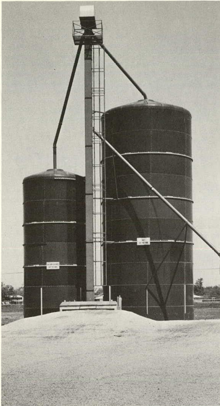
CHEMICAL STORAGE SILOS FOR PROVIDING VARIABLE MIXES.
