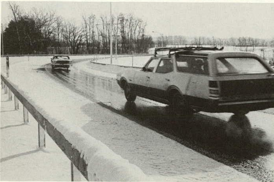
Figure 1. Cross-pavement drainage of snowmelt.
