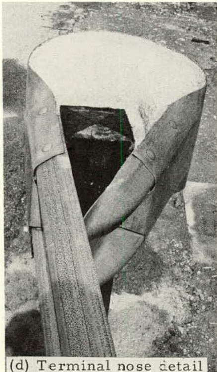
Figure A-21. Installation details, Test 130.
