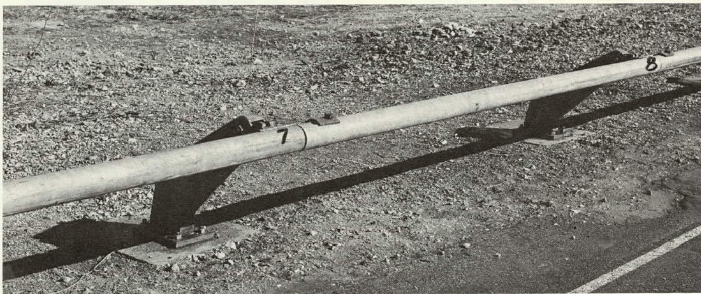
(b) Close-up of Test 129 Installation
