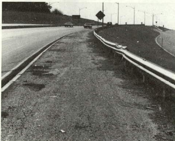
Figure 8. Accident involving curb and guardrail.
