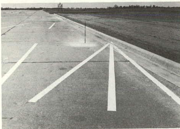
Type C Curb in Foreground
