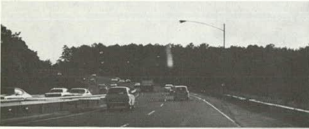
I85 SOUTHBOUND, 4 LANE, DIVIDED FACILITY, NO ENVIRONMENTAL BUILDUP, 400 WATT CLEAR MERCURY VAPOR ILLUMINATION SYSTEM AT 30FT. MOUNTING HEIGHT.
