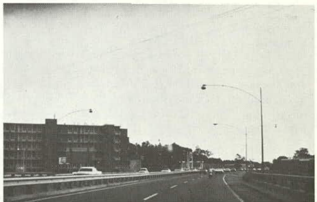
I85 SOUTHBOUND TYPICAL SECTION WITH HEAVY ENVIRONMENTAL BUILDUP.
