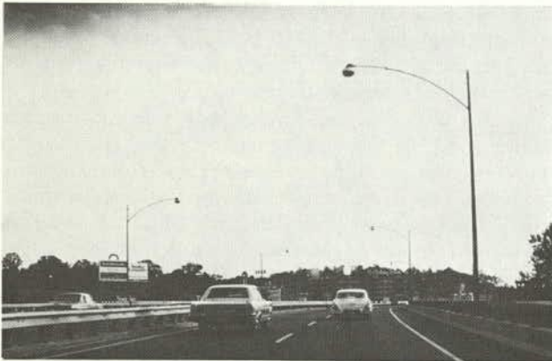
I85 SOUTHBOUND ELEVATED SECTION, STAGGERED ILLUMINATION CONFIGURATION.
