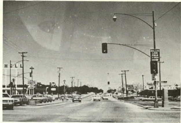
TYPICAL SECTION OF UNLIGHTED PORTION OF NORTHWEST HIGHWAY. SAFETY LIGHTING IN USE AT ALL MAJOR INTERSECTIONS.
