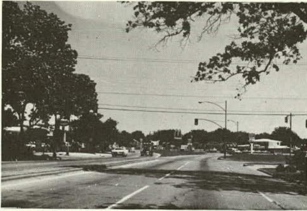
INTERSECTION OF NORTHWEST HIGHWAY WITH BACHMAN LANE, FOUR-LANE DIVIDED, BEGINNING OF HEAVY ENVIRONMENTAL BUILDUP.
