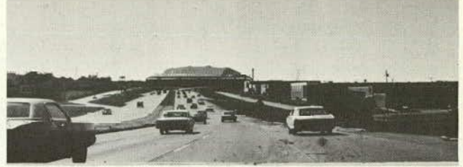
END OF ELEVATED SECTION APPROACHING WYE OF US 183 AND US 114 NORTHBOUND. LITTLE ENVIRONMENTAL BUILDUP.
