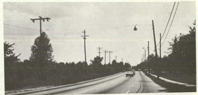
PEACHTREE ROAD SOUTHBOUND, ONE-SIDED ILLUMINATION SYSTEM, 400 WATT CLEAR MERCURY VAPOR AT 30 FT. NO SHOULDER, UNEQUAL LANE WIDTH.
