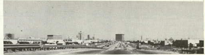
END OF ELEVATED SECTION OF US 183, SOUTHBOUND APPROACHING URBAN AREA. HEAVY ENVIRONMENTAL BUILDUP.
