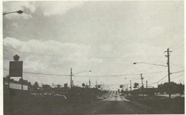
PEACHTREE ROAD SOUTHBOUND, TYPICAL SECTION, HEAVY ENVIRONMENTAL BUILDUP.
