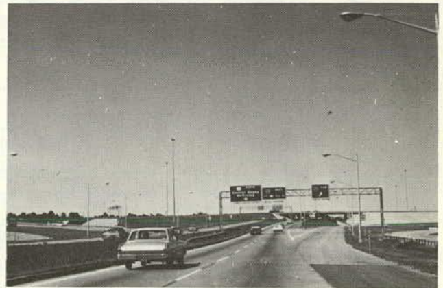
INTERCHANGE OF US 75 WITH I 635 OF PARTIAL CLOVERLEAF TYPE. ILLUMINATED WITH HIGH-MAST SYSTEM.
