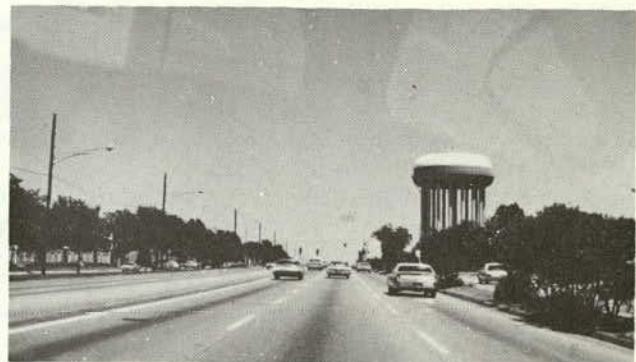
ONE SIDED ILLUMINATION SYSTEM, 400 WATT CLEAR MERCURY VAPOR AT 30FT. NO SET SPACING. BEGINNING OF HEAVY ENVIRONMENTAL BUILDUP.
