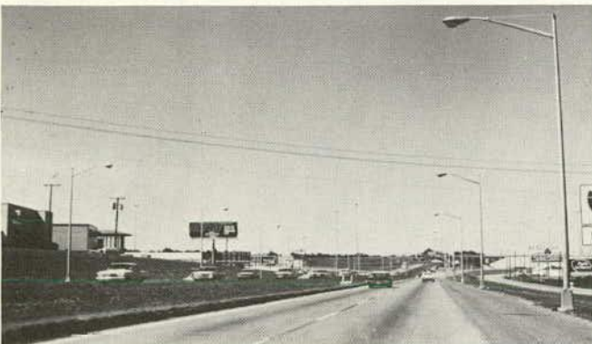
US 75 NORTHBOUND, APPROACH INTERCHANGE WITH I 635 FOUR-LANE DIVIDED, WITH NO MEDIAN BARRIER. 400 WATT CLEAR MERCURY VAPOR ILLUMINATION SYSTEM @ 30 FT.
