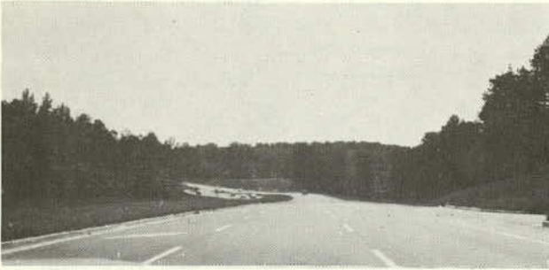
INDUSTRIAL BLVD., SOUTHBOUND, FOUR-LANE DIVIDED ROADWAY, NO ENVIRONMENTAL BUILDUP.
