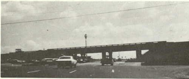
INTERCHANGE OF INDUSTRIAL BLVD. SOUTHBOUND & I 285, APPROACHING PEACHTREE ROAD.
