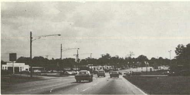
PEACHTREE ROAD SOUTHBOUND, ONE-SIDED ILLUMINATION SYSTEM, 400 WATT CLEAR MERCURY VAPOR AT 30 FT.
