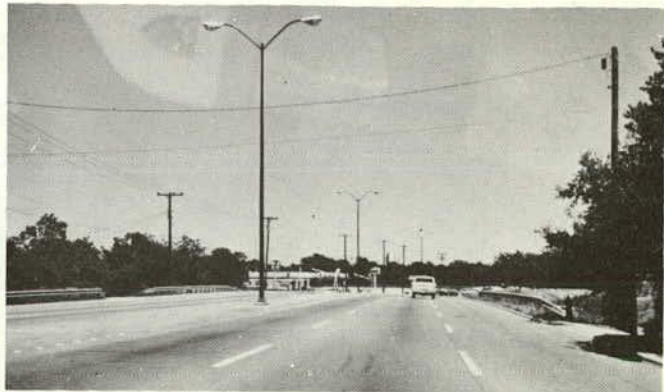
VIEW OF SAME FACILITY, APPROACHING 1ST SIGNALIZED INTERSECTION. VERY LITTLE ENVIRONMENTAL BUILDUP.
