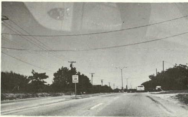
BEGINNING OF ILLUMINATED SECTION, CHANGES FROM 2 LANE UNDIVIDED TO SIX LANE DIVIDED, LIGHTING SYSTEM CLEAR MERCURY VAPOR, 1000 WATT AT 40FT., 250FT. SPACING.
