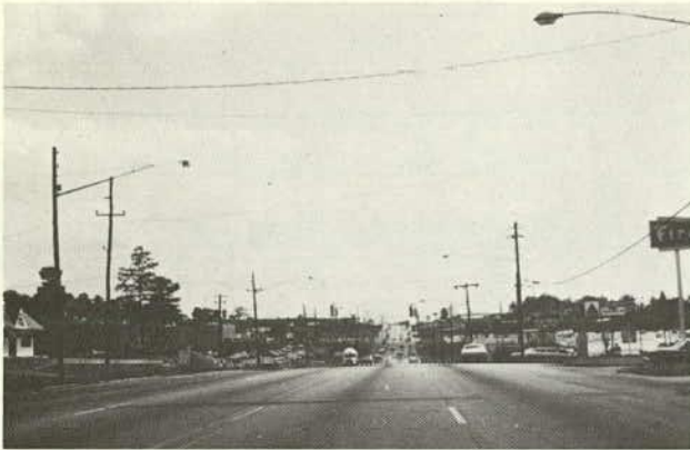
PEACHTREE ROAD SOUTHBOUND, FOUR-LANE UNDIVIDED, STAGGERED ILLUMINATION SYSTEM, 400 WATT CLEAR MERCURY VAPOR AT 30 FT; SPACING VARIABLE, MOUNTED ON EXISTING UTILITY POLES.
