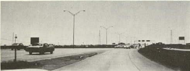
MERGE OF INWOOD DRIVE ENTRANCE RAMP WITH I 635 EASTBOUND. EIGHT-LANE FACILITY. 1000 WATT CLEAR MERCURY VAPOR SYSTEM AT 50 FT, 250 FT SPACING.
