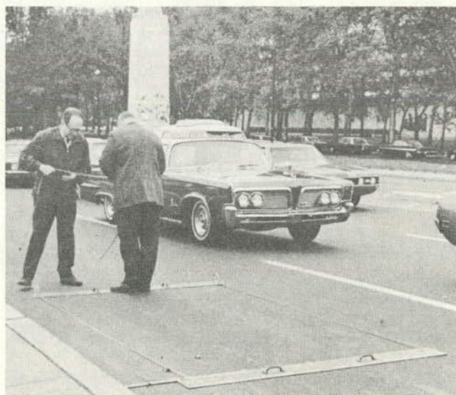
Figure 6. Measuring boards used to position Tapeswitch detectors.
