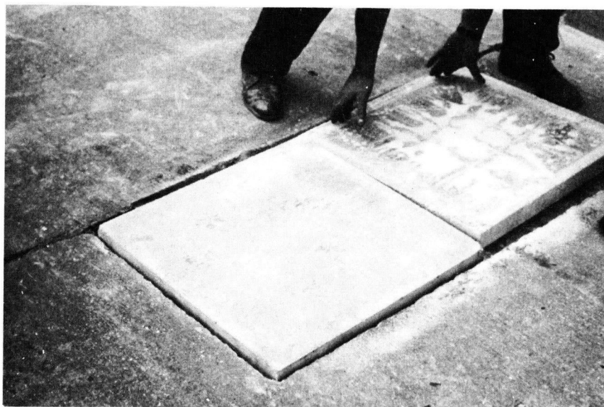
Figure 10. Two-inch-thick precast slabs used as a partial-depth concrete patch.
