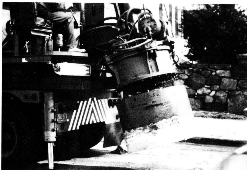
Figure 11. Cylindrical saw used to make full-depth utility cuts in concrete pavements.
