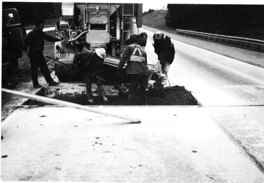
Figure 14. Custom-sized concrete batches being supplied by special concrete mixing truck.
