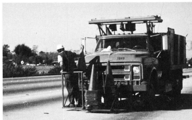
Figure 7. Truck-mounted safety platform used in manual placement of traffic control cones.
