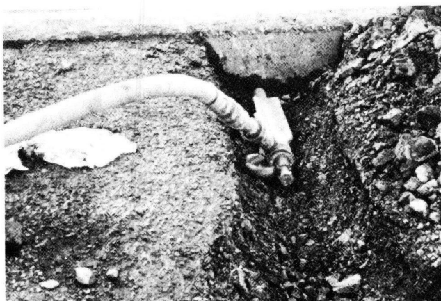
Figure 16. Horizontally driven pipe used to pump slurry under pavement slab in mudjacking operation.
