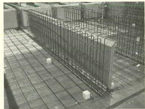
Fig. E-32 Girder Reinforcement and Formwork for Specimen SC-3
