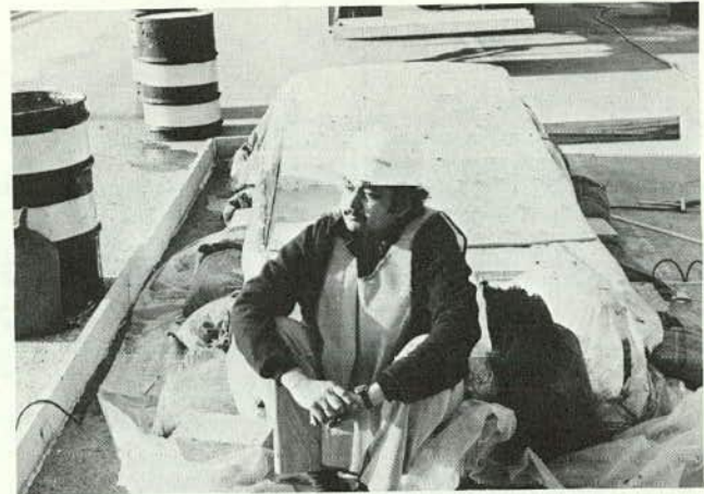
Figure H-31. Close-up of insulated chamber.
