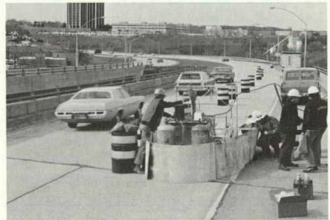
Figure H-20. Drying in progress.
