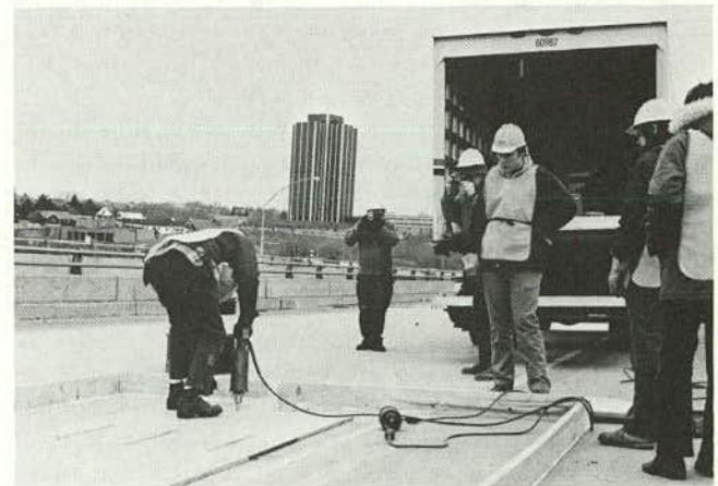
Figure H-26. Drilling bolt holes for impregnation unit.
