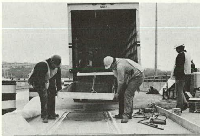
Figure H-28. Placement of chamber over gaskets.
