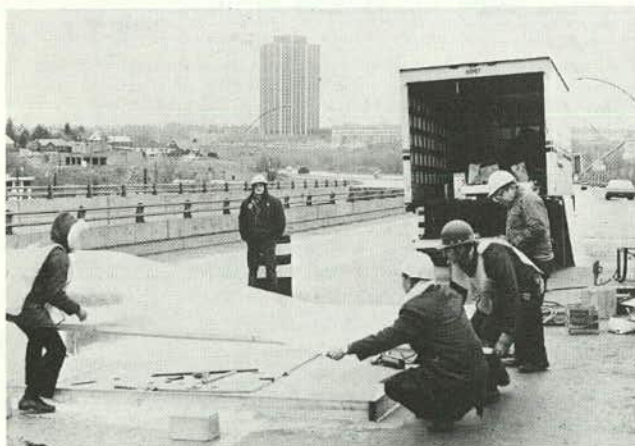
Figure H-25. Covering of working area against rain.
