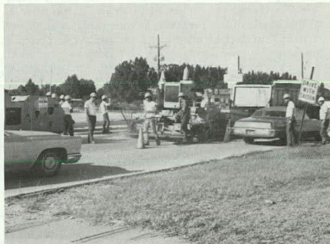
Figure F-1. Paving operations with traffic US 50.
