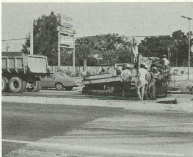
Figure 1. Paving operations on US 50 at SR 436.
