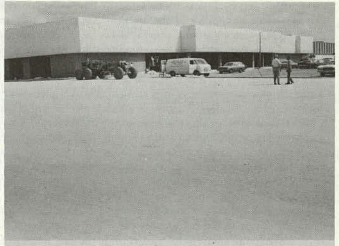
Figure F-4. Shopping center parking lot, looking NE—Altamonte Springs, Fla.
