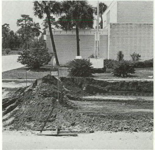
Figure E-20. Field location #3—construction south of samplers.
