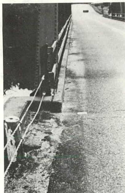
Figure A-14. Photos of Seabastick Bridge (truss bridge).
