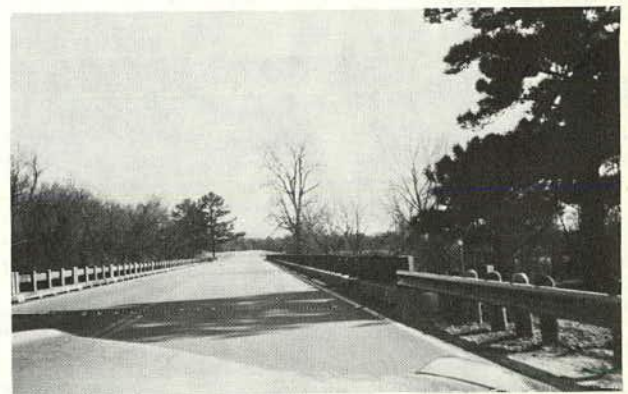
U.S. 77 (View of bridge rail) La Grange
