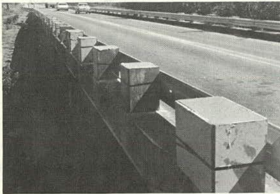
Figure 14. Tops of broken concrete posts formed and concrete poured.
