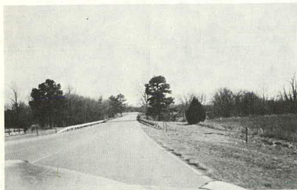
U.S. 77 (View of approach guardrail) La Grange
