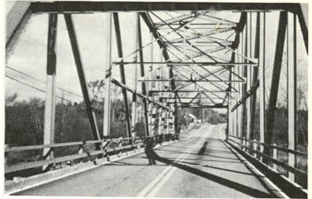
(b) Treatment No. 1 (edgeline on bridge)
