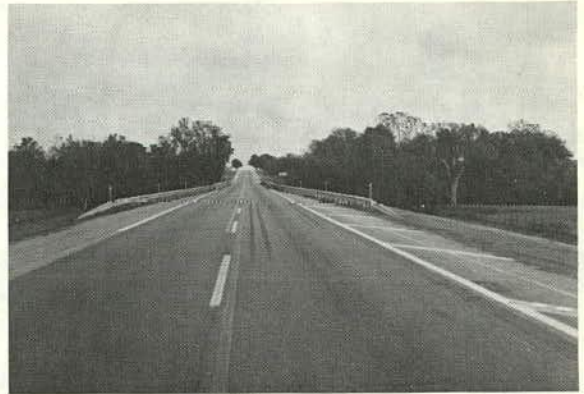
Figure 15. Completed project picture shows flex-beam rail across bridge with approach rail attached.
